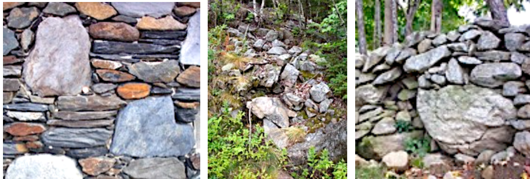
Left to right: Patterned degree of order that is above and beyond a laid degree of order. Cliff Walk, RI. Dumped degree of order in a stone band, Weld, ME. Stacked degree of order in Hebron, CT.
