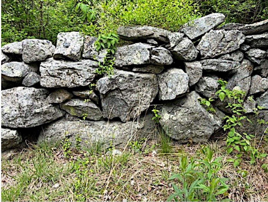
Jagged blocks of Avalonia granite hefted and stacked onto a single wall in Stonington, CT. Only one tier is present and no courses. The largest stone at base is of the Assisted size category.
